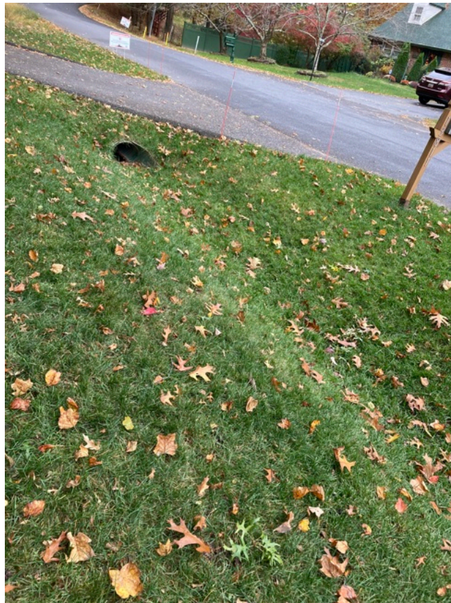
A.4 Drainage ditch and conveyance pipe under driveway of 13811 Shannon Drive.
