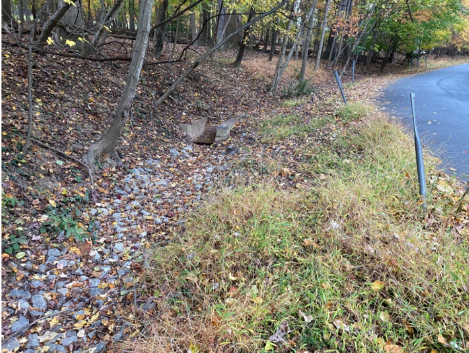
A.3 Drainage ditch and drain to conveyance pipe under Shannon Drive
