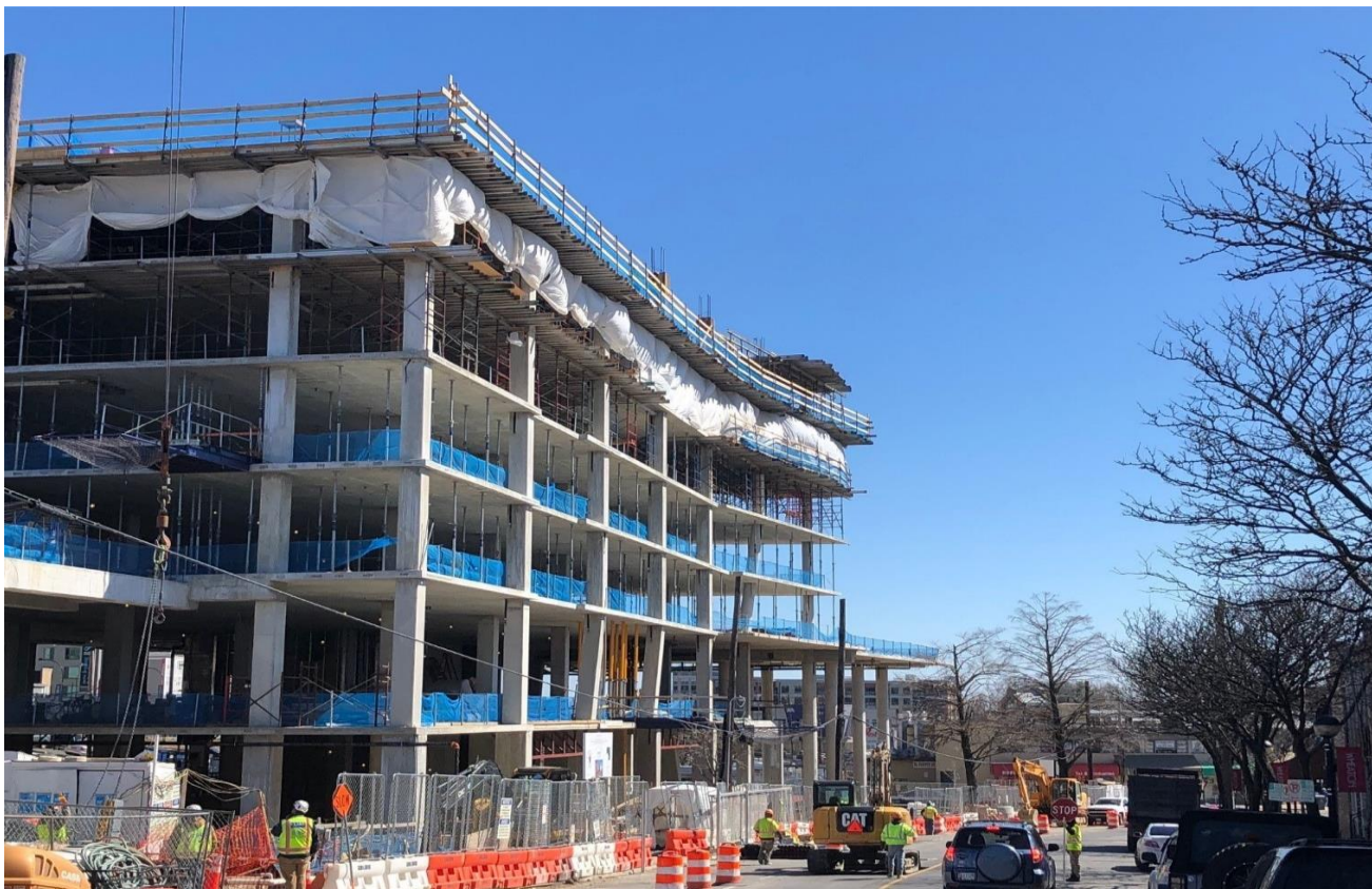
Eighth floor under construction - March 28, 2019
