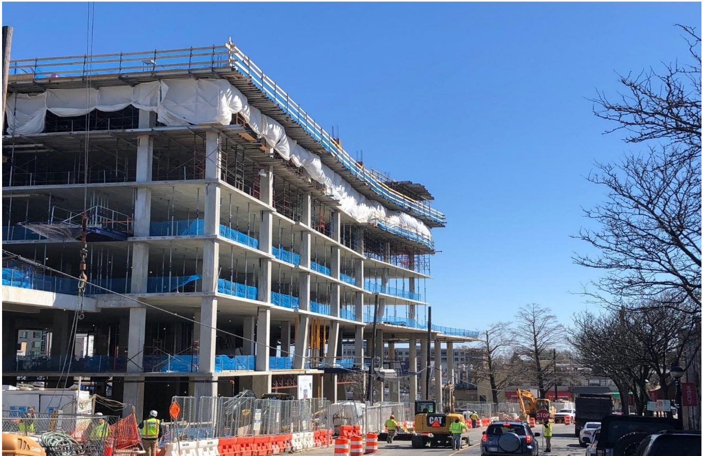
Eighth floor under construction - March 28, 2019
