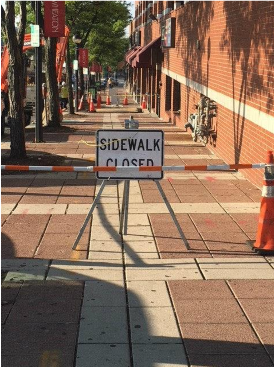
New Pepco Vault being constructed in sidewalk along Grandview Avenue
