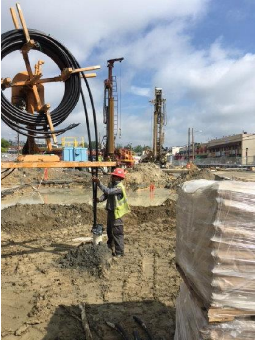
Installing the Geothermal Tubing 650-feet Into the Borehole (August 18, 2017)
