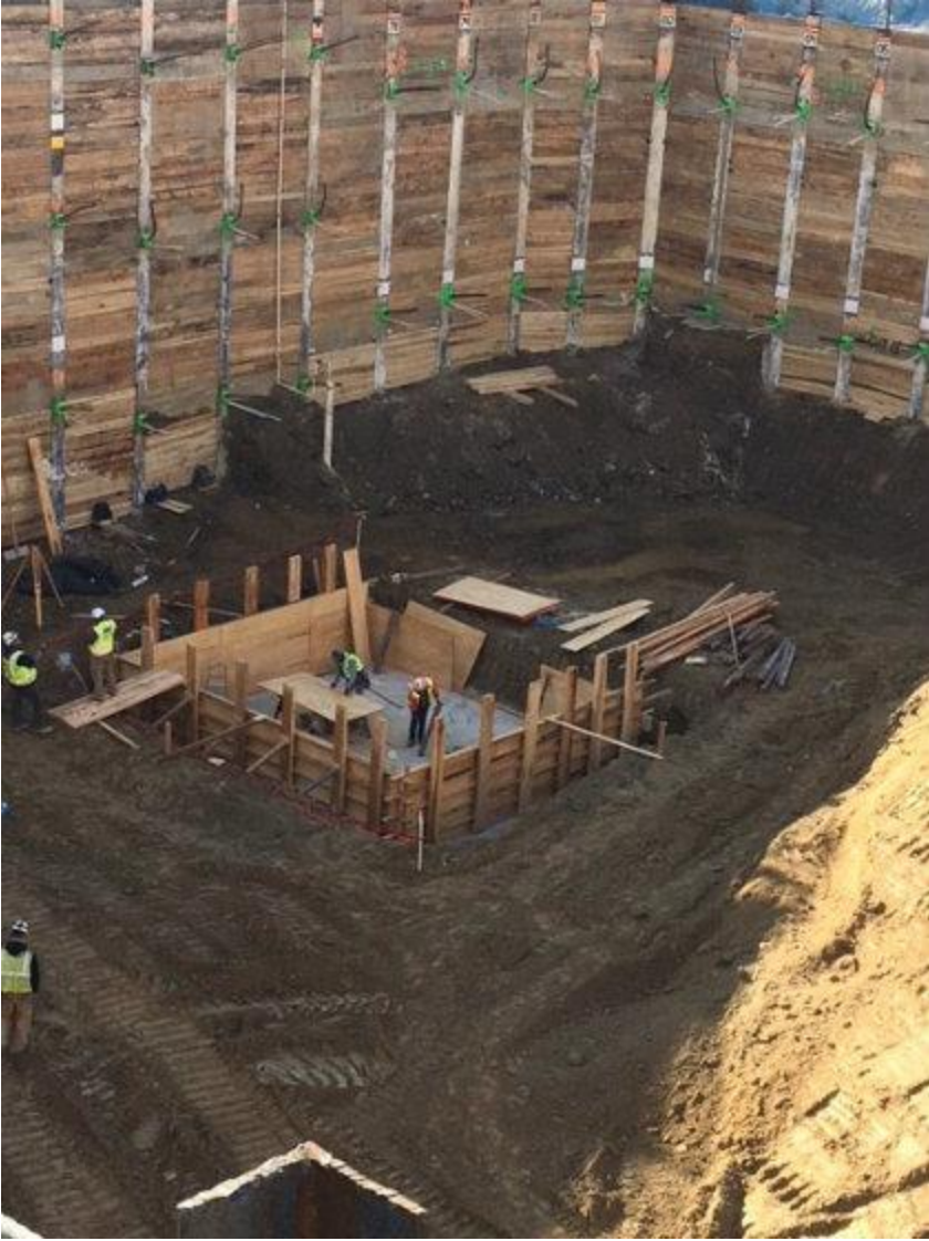
South Tower Crane Foundation
