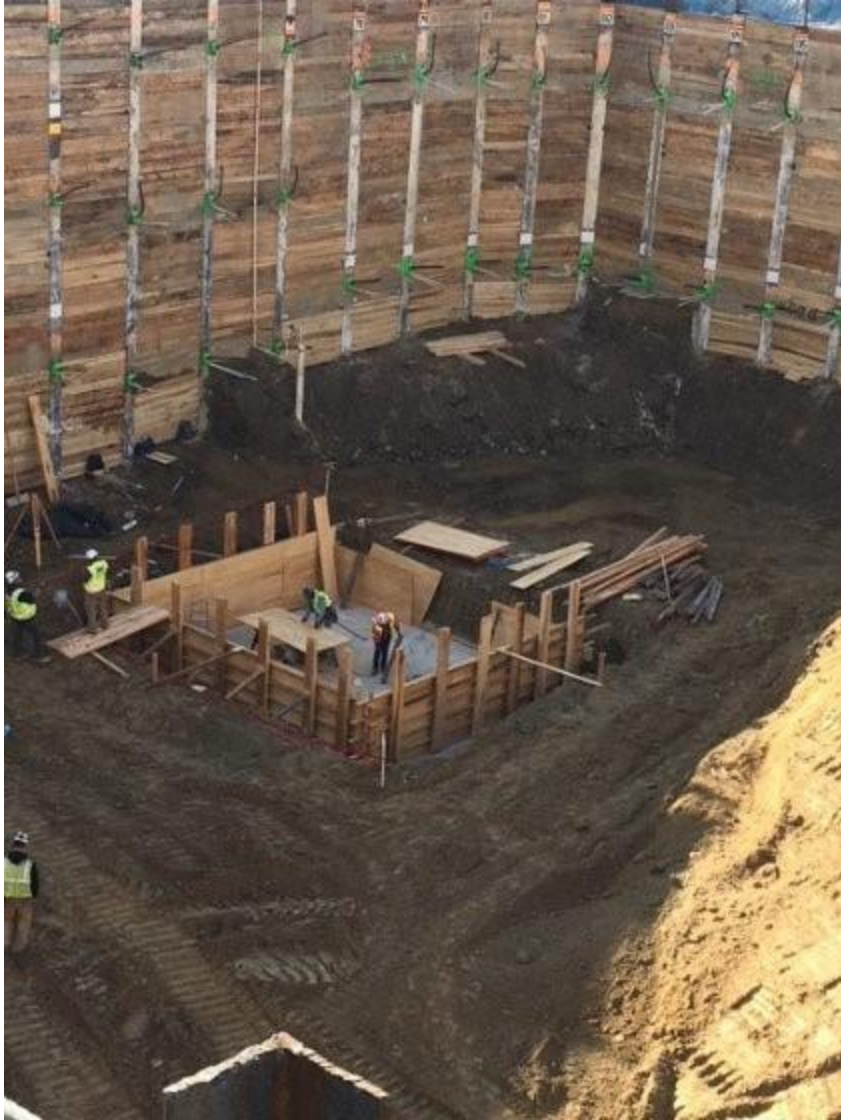
South Tower Crane Foundation
