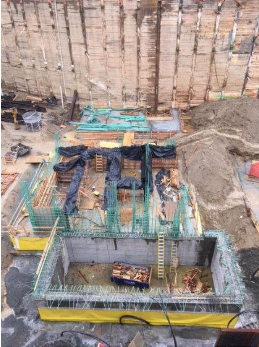
Area Below Main Lobby & Elevators
