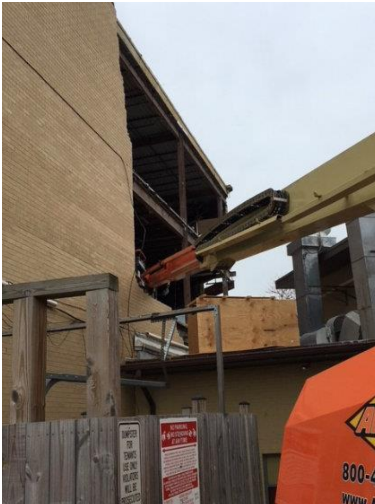
Demolition of the northernmost wall of the Regional Services Center (RSC)
