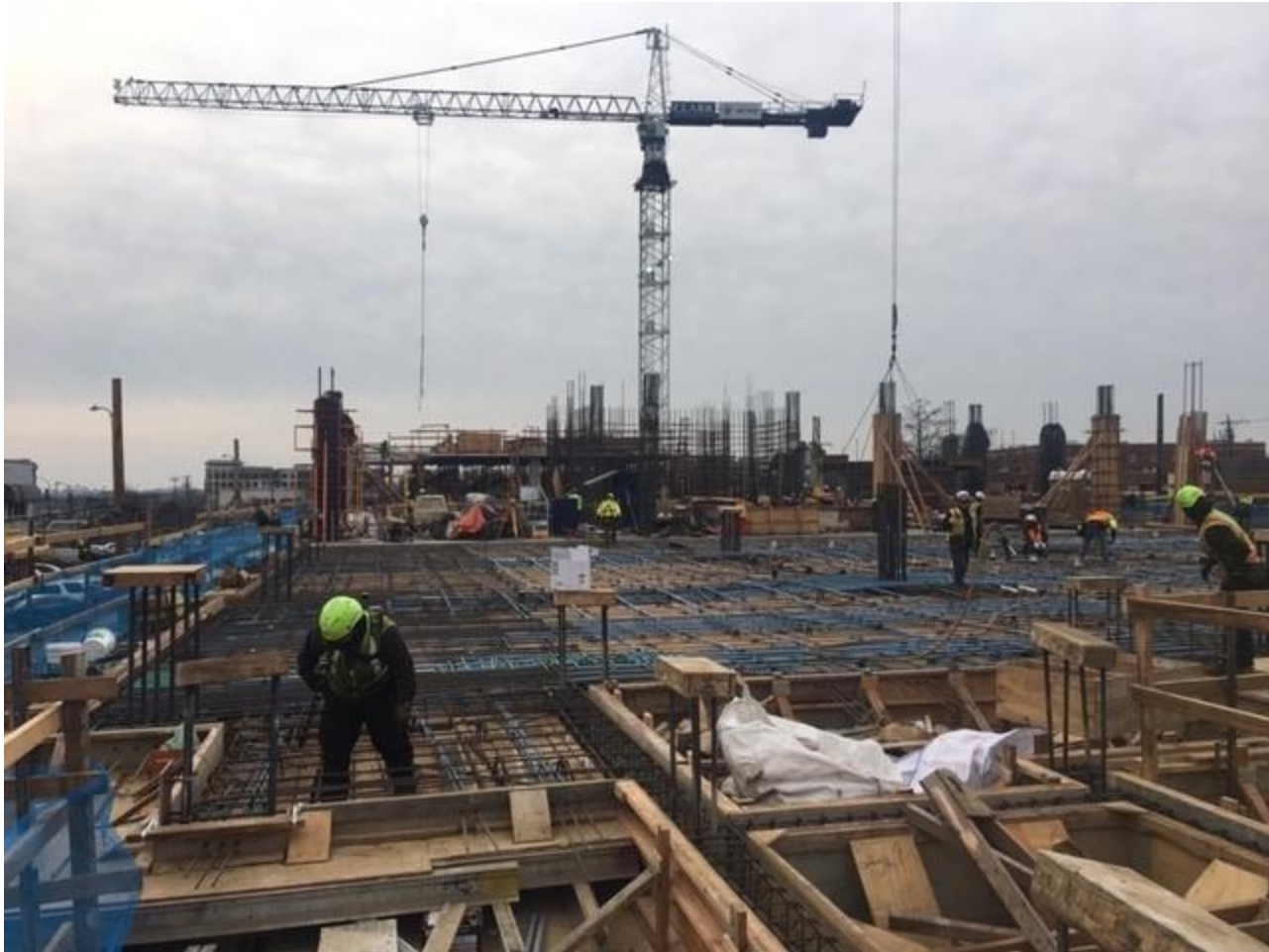
January 2019 - Photo showing second-floor (foreground) third-floor (background)
