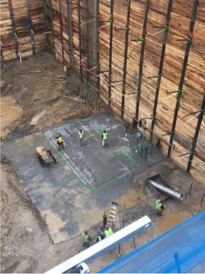
Foundation for north tower crane under construction
