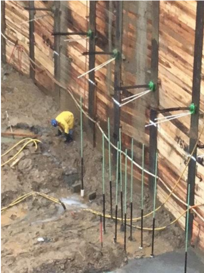
Embedded tie-down anchors at the north end of the site
