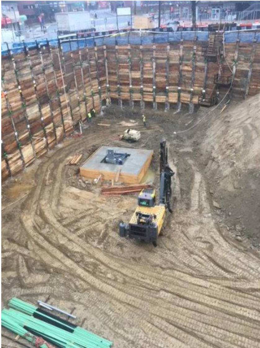
South tower crane foundation
