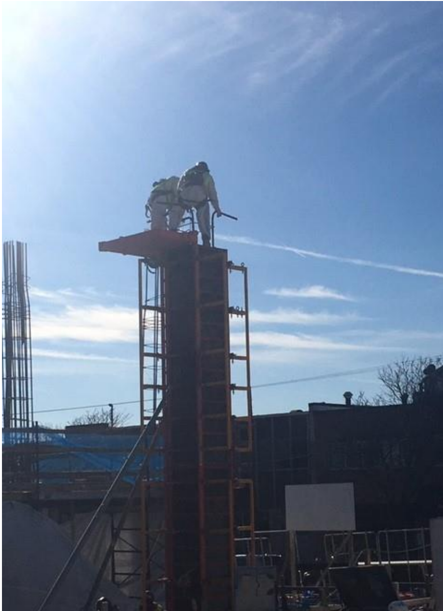
Column Construction Underway - January 10, 2019
