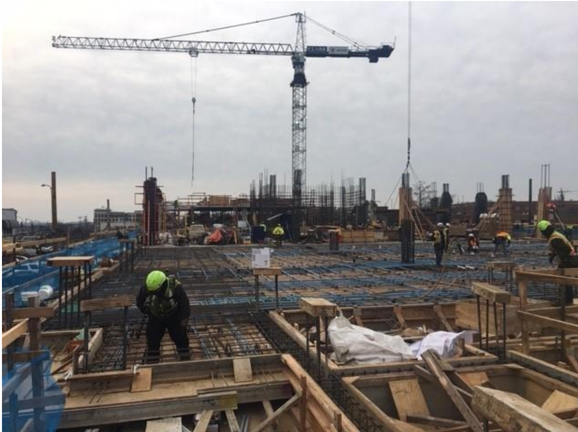
Photo showing second-floor (foreground) third-floor (background) - January 10, 2019
