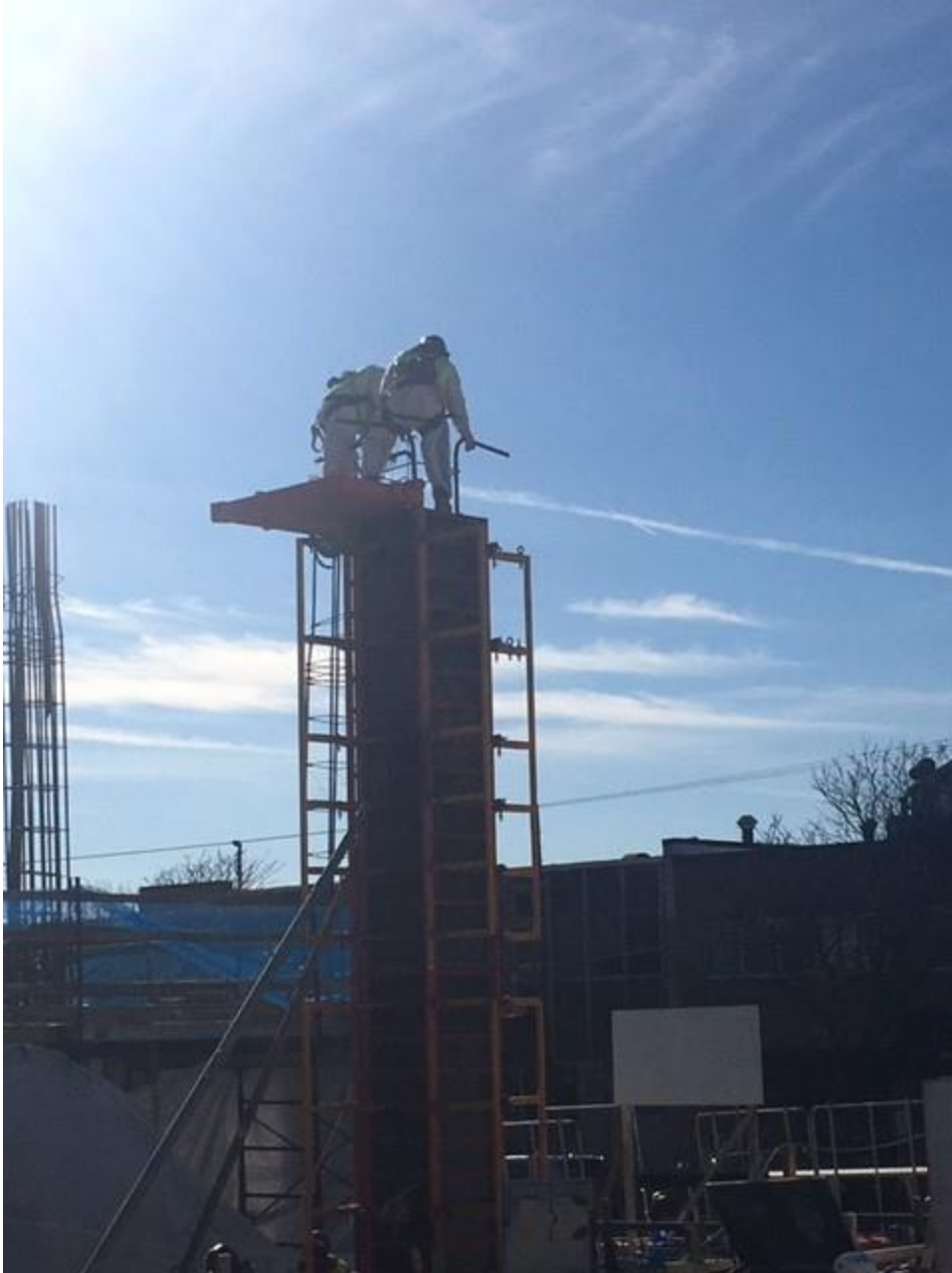
Column construction underway
