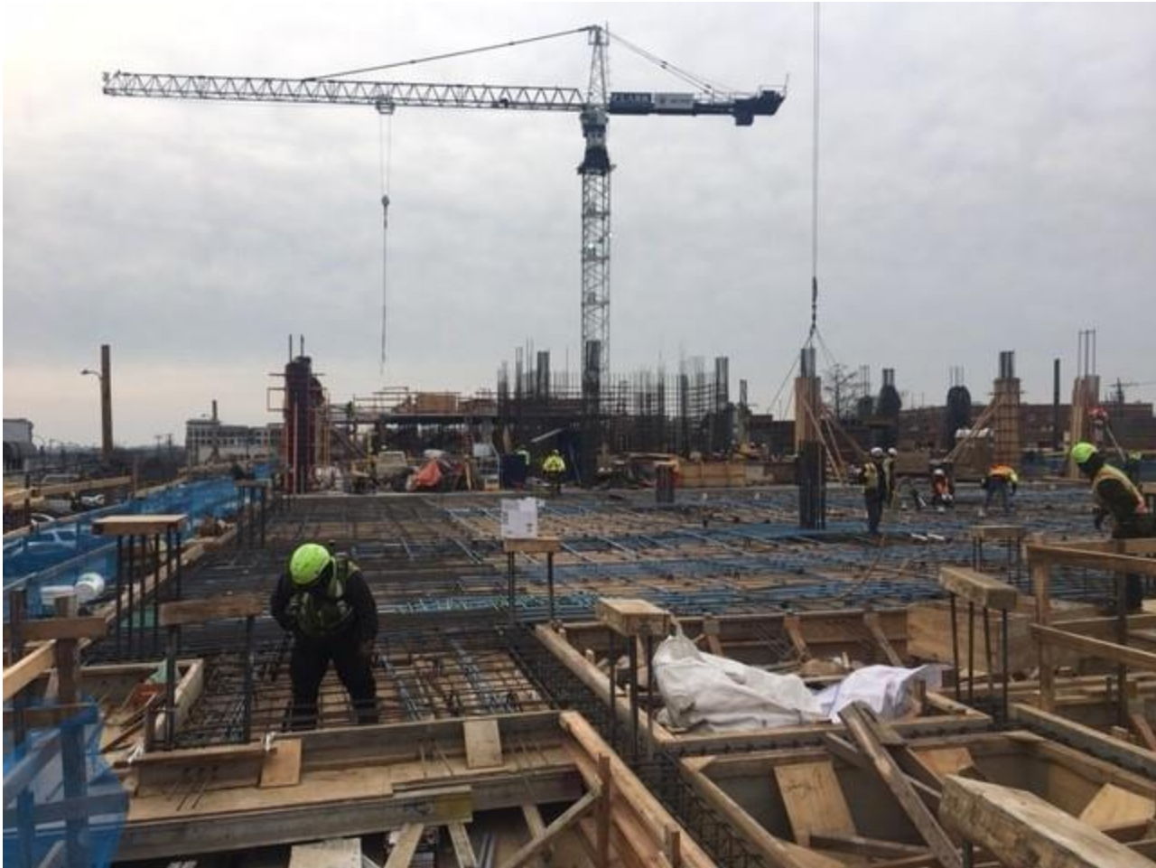
Photo showing second-floor (foreground) third-floor (background)
