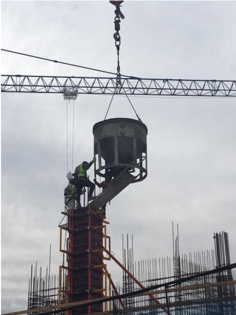
Photo showing column pour between the second and third floors
