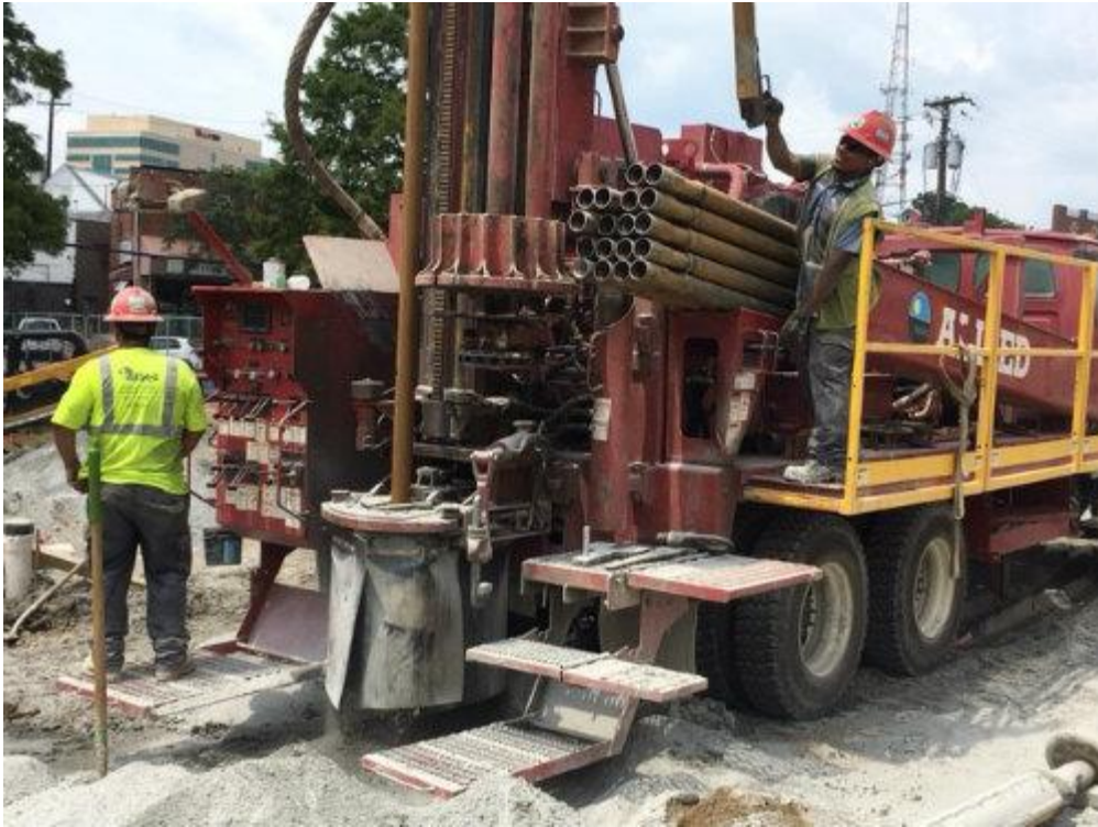
Typical Drill Rig
