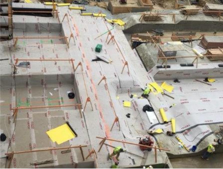
The bottommost floor level of the parking garage (known as P-4) will be placed atop the waterproofing system, as shown above.
