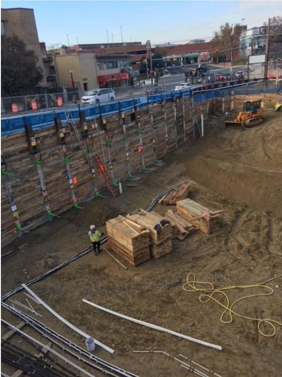
Excavation Advances along Triangle Lane
