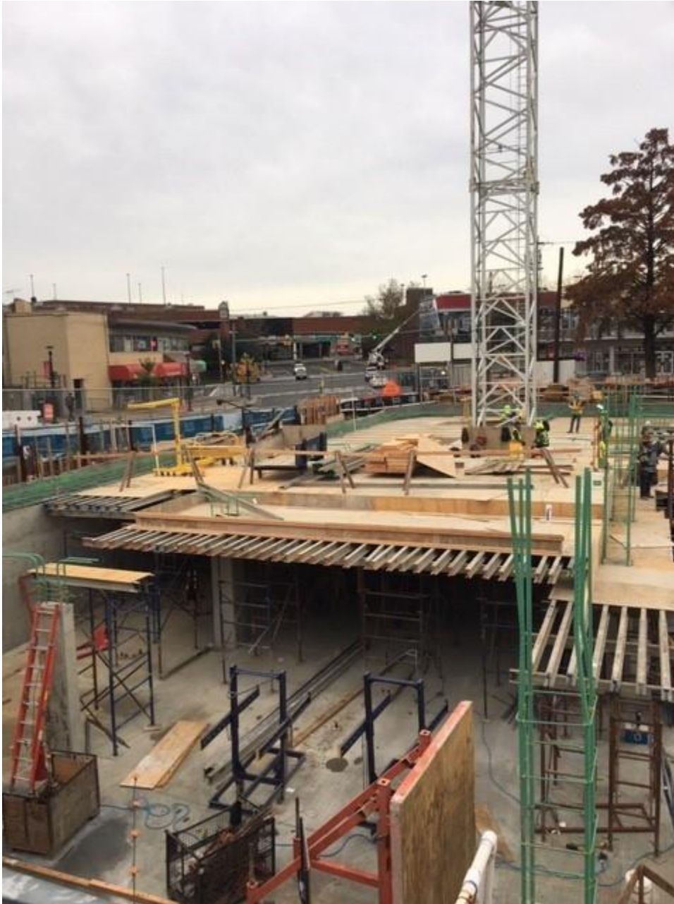
Garage Level P0 reaches street level at Reddie Drive
