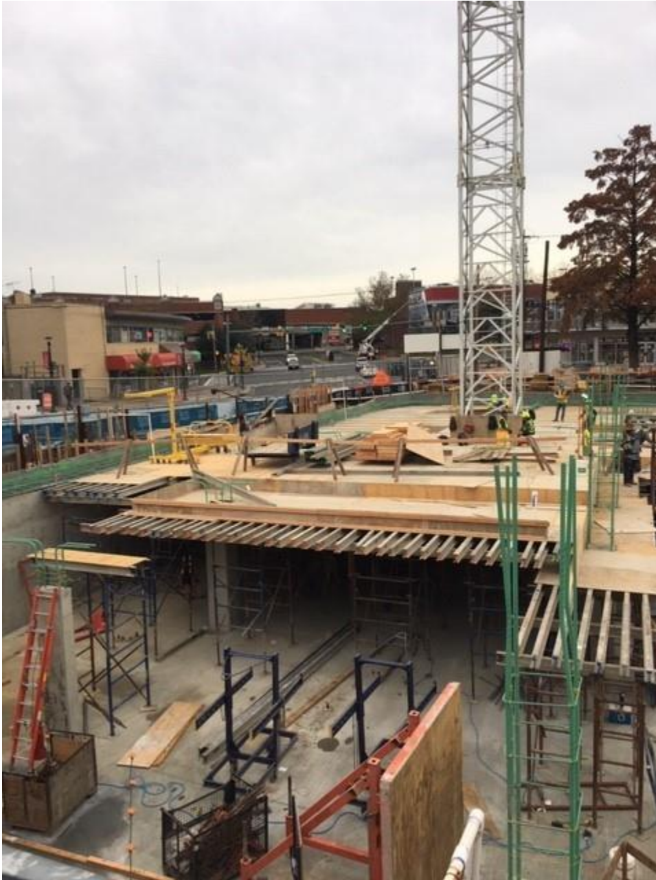
Garage Level P0 at Reddie Drive
