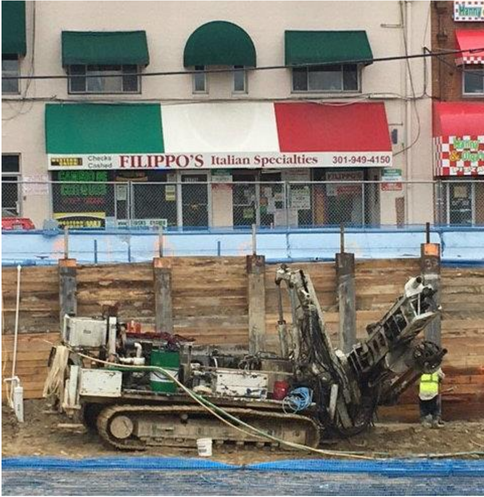
Tie Back Anchor Machine
