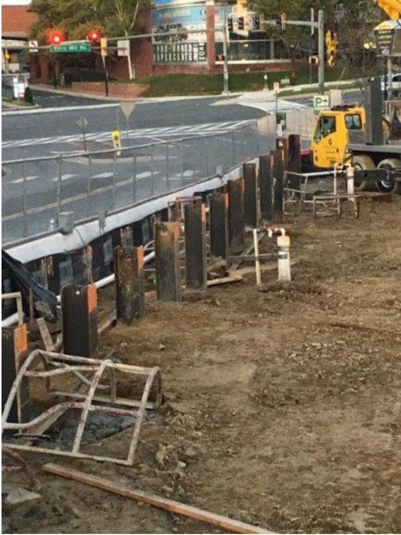
First Row of Soldier Piles Installed - September 8, 2017
