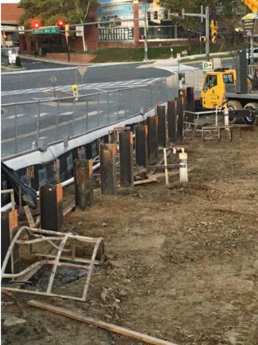
First Row of Soldier Piles Installed - September 8, 2017
