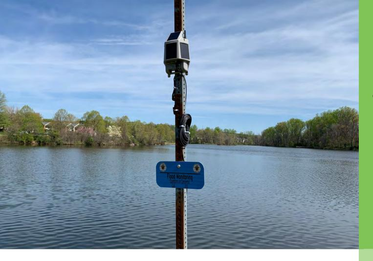
A total of 35 flood sensors were installed at the County's frequently flooded sites, providing real-time data to various agencies and jurisdictions, enhancing flood response and management.
