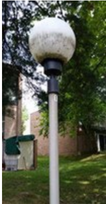
Montclair Manor Community Streetlight Before
