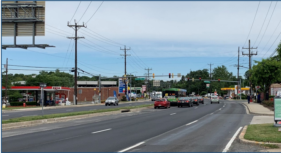
Figure 6-1: Existing Intersection of MD 650 and Powder Mill Road from the South
