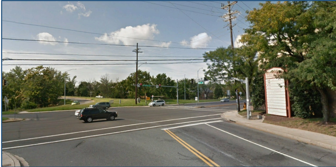
Figure 6-3: Existing Intersection of MD 650 and Elton Road from the East
