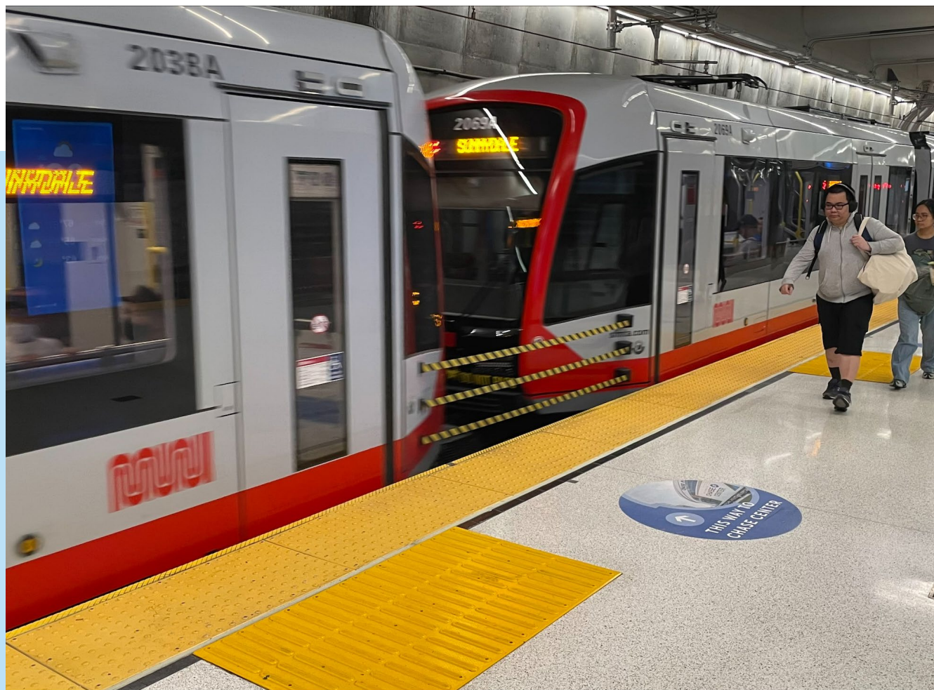
Figure 15: Example of transit door location TDIs
