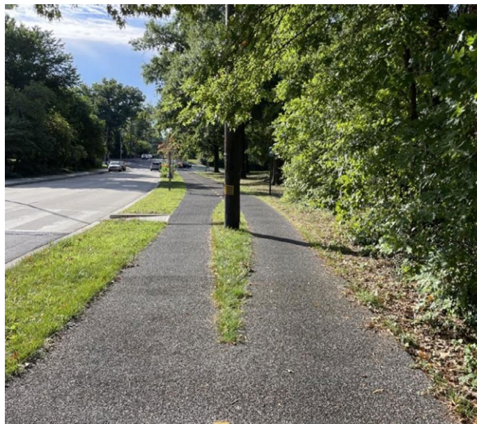
Figure 21: A shared use path splits around a utility pole. The wedge of grass provided is a non-prepared surface that may help people with vision disabilities navigate around the obstacle. Retroreflective edge lines could also be used to help define the correct path in this context.
