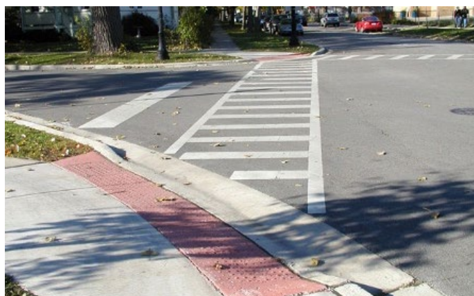
Figure 37: Example of curb ramp that is not aligned with crosswalk.
