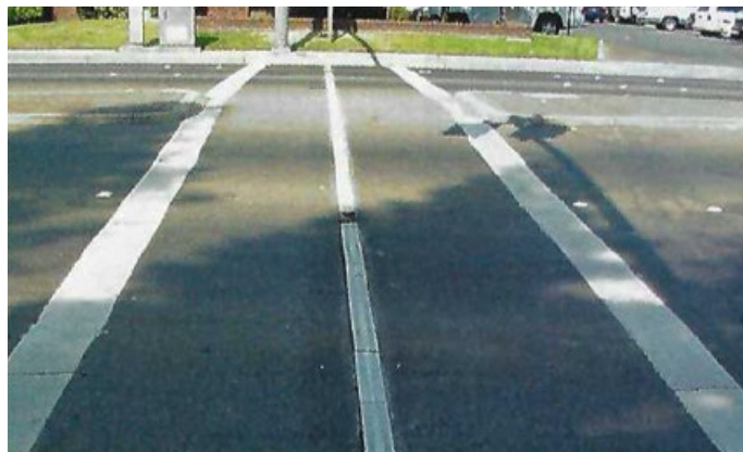
Figure 65: Sacramento crosswalk guide strip example from report conducted by the Sacramento Department of Public Works.
