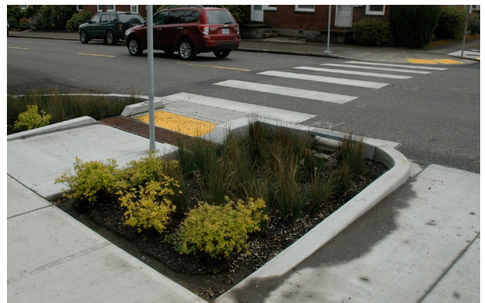
Figure 42: Parallel curb ramp example
