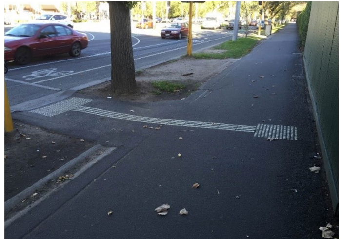
Figure 32: Example of tactile direction indicator used to guide pedestrians with vision disabilities to a midblock crosswalk in Melbourne, Australia. Note that the bars are not oriented as specified in this guide for sidewalk alert TDIs.
