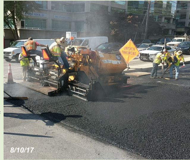
Crews laying new asphalt at Spring Street and Georgia Ave.
