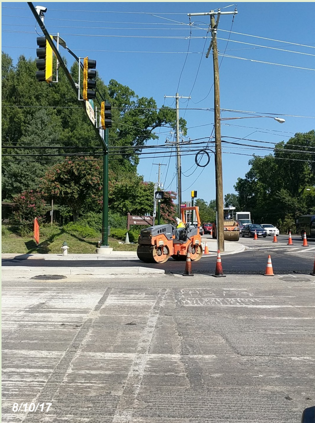
Left: Milling complete in the foreground, paving underway in the background. Right: Completed paving on Spring Street between Second Ave and First Ave.
