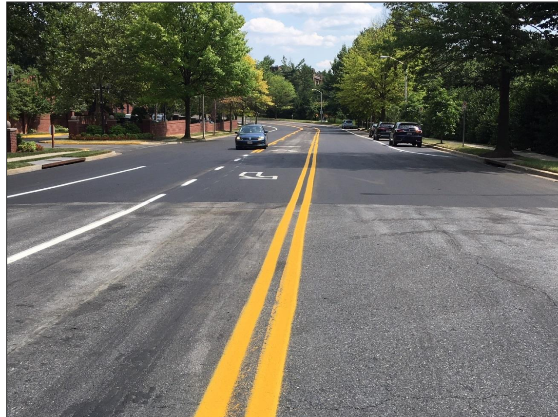
Existing Executive Boulevard looking south from Nicholson Lane
