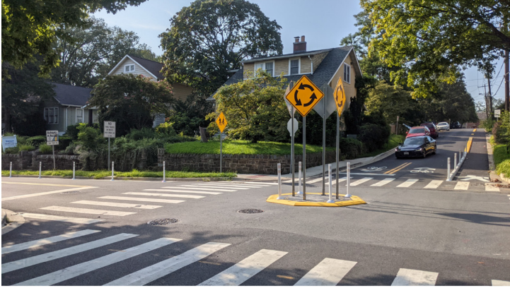
Above image: mini-roundabout at Silver Spring Avenue.
