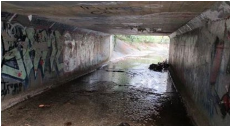
Cell 1 (looking north)
