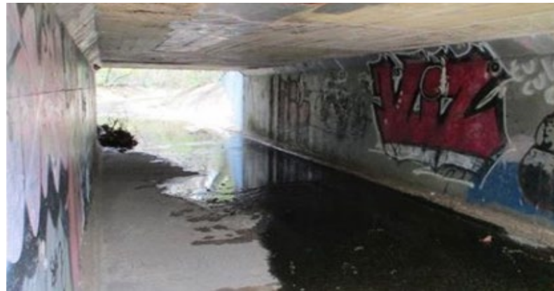
Cell 2 (looking north)
