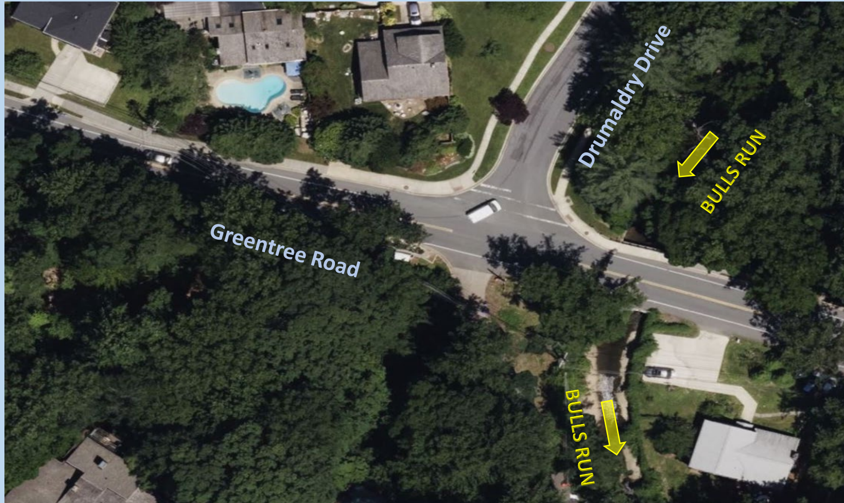
Aerial View – Greentree Road Bridge No. M-0180
