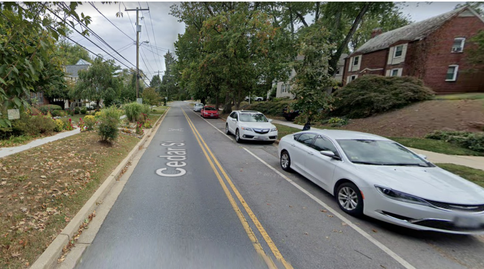
Above: existing condition on Cedar St
