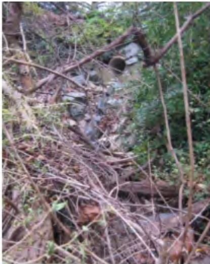
Figure 3B.1 Pipe Outfall
