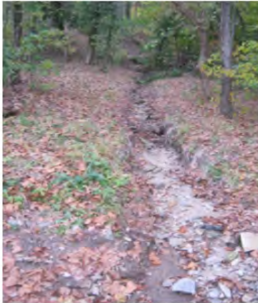
Figure 2.1 Ditch Erosion
