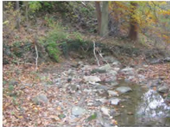
Figure 1A.2 Bank Erosion
