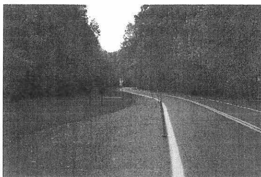
Figure I-9: Flex Posts Installed to Separate Bikeway and Roadway
