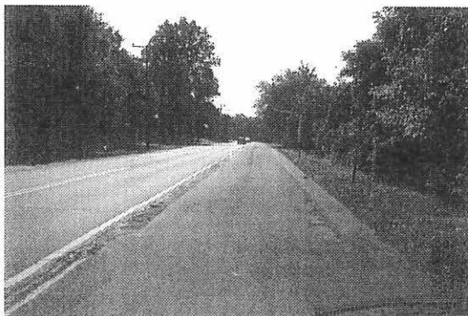
Figure I-3: Substandard Shared Use Path (Not Separated from Roadway)
