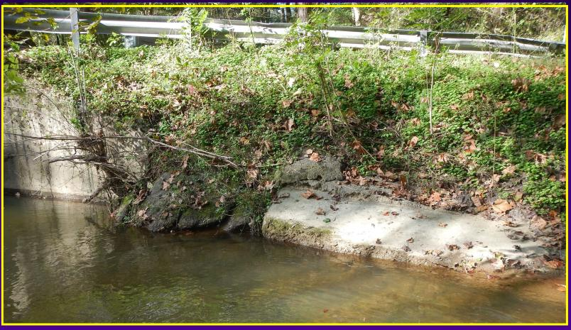
■ Failed concrete and asphalt streambank protection
