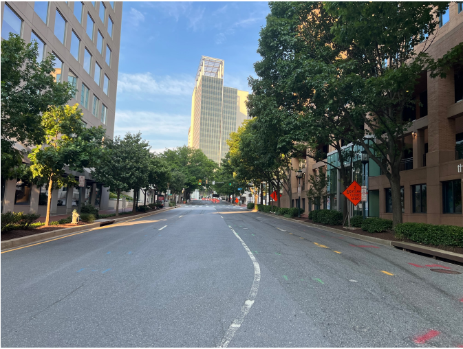
Existing Conditions looking East along Montgomery Lane
