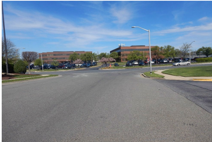
Photo 16 – Absent Lane Markings on East Approach
