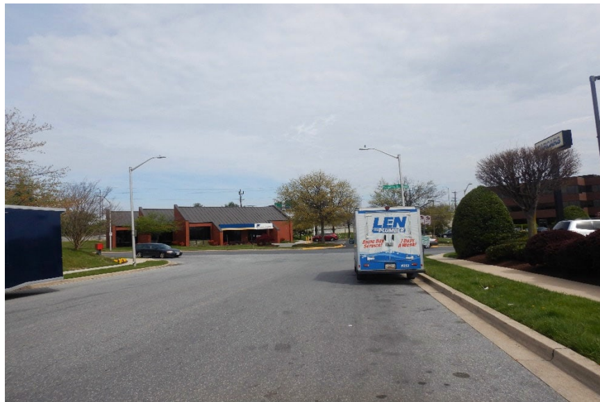
Photo 15 – Absent Lane Markings on East Approach
