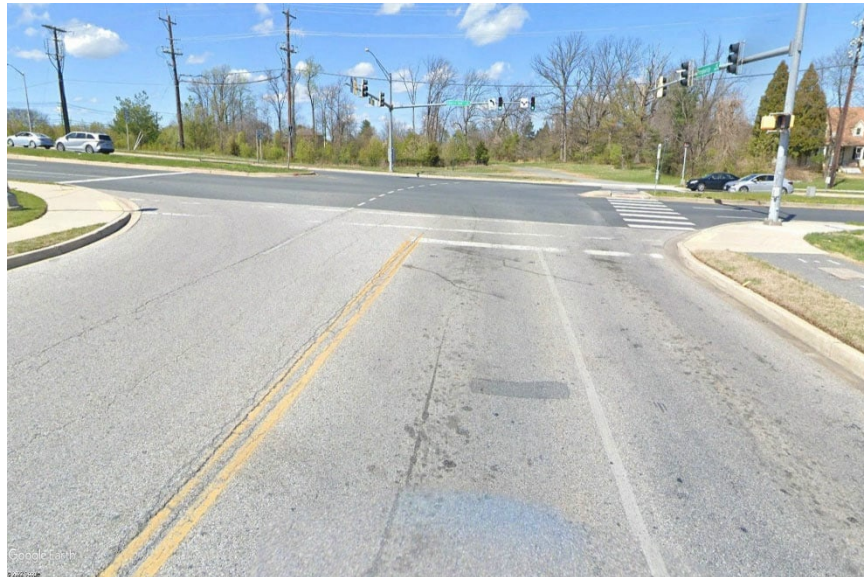
Photo 7 – Study Intersection 6: Prosperity Drive at Cherry Hill Road (Looking North)
