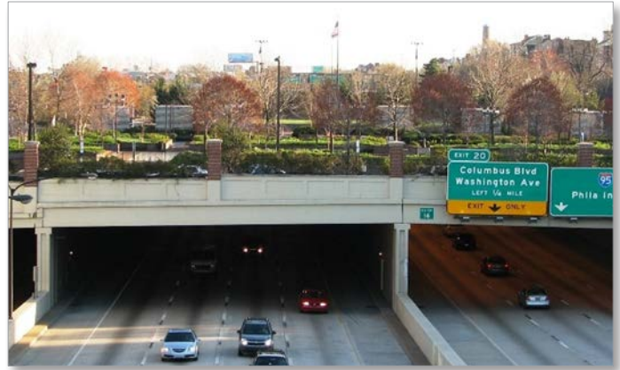
I-95 bridge with trees and landscaping in Philadelphia, PA
