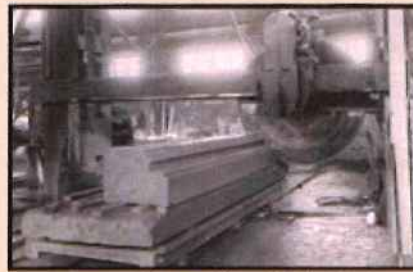
Large stone-cutting machine at Fuller Plant (Source: Washington National Cathedral Archives)
