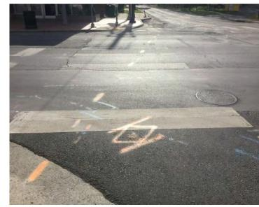
Figure 8-14 Faded and missing crosswalk striping at the intersection of Fenton Street and Silver Spring Avenue.
