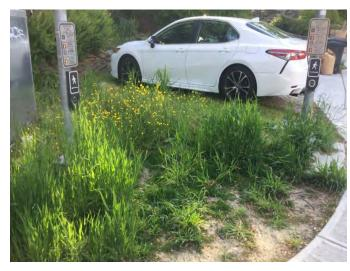
Figure 8-11 This crossing needs to have its pushbutton relocated because it is not near the sidewalk.
