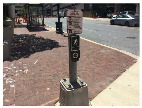
Figure 7-16 APS unit does not make an audible sound when activated
