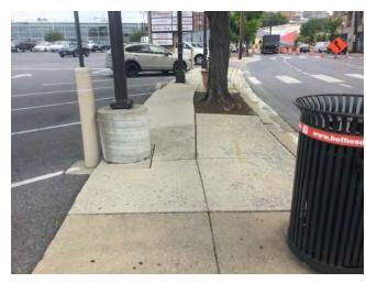
Figure 3-11 A noncompliant sidewalk slope on Arlington Road.
