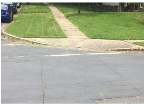
Figure 11-5 A non-compliant curb ramp.
