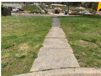
Figure 9-4 Mismatched and broken portion of existing sidewalk.
