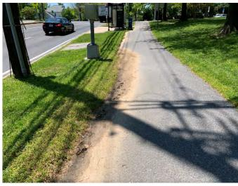
Figure 2 -19: Drainage issues cause sediment buildup.
