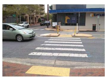
Figure 3-6The median opening is too narrow.
