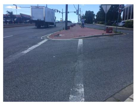
Figure 13-11 Non-compliant Curb Ramp.
