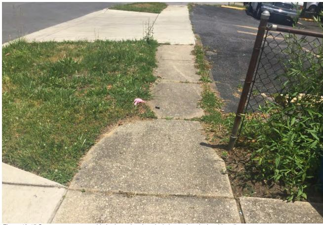
Figure 13-15 Overgrown grass provide horizontal and vertical obstructions in the sidewalk.
