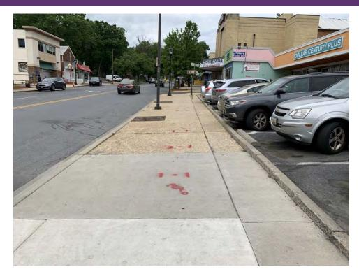
Figure 11-10 Sidewalk with non-compliant slope along Flower Avenue.
