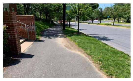
Figure 7-22 Soil erosion on to shared use path along Colesville Road.
