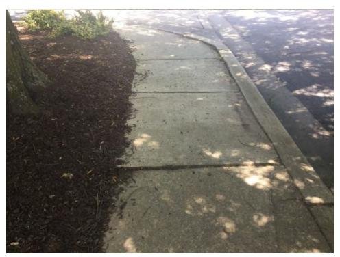
Figure 13-5 Vertical Tripping Hazard.
