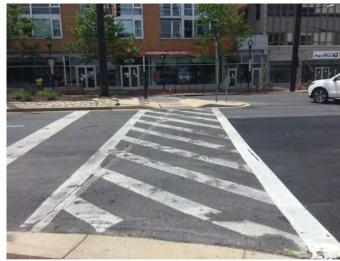
Figure 3-4 A typical crosswalk with outdated markings
