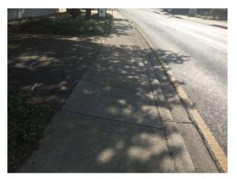
Figure 3-12 A non-compliant driveway apron on Montgomery Avenue.
