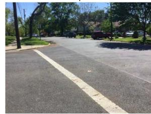
below; the crosswalk along Spencer Road should be restriped and an additional curb ramp should be constructed at the intersection shown.
