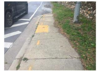
Figure 4-14 Existing curb ramp along Jones Bridge Road does not have an adequate landing area.
