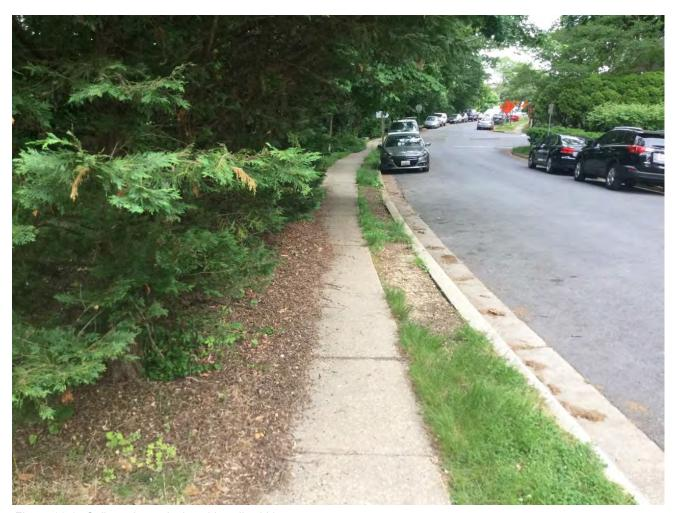
Figure 11-15 Soil erosion reducing sidewalk width.
