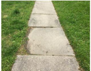
Figure 6-4 Broken portion of existing sidewalk.
