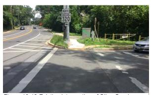
Figure 10-13 Existing intersection of Sligo Creek Parkway and Piney Branch Road (MD 320) with lacking APS/CPS..
