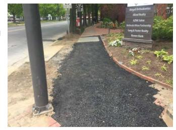
Figure 3-2 Asphalt utility patching at intersection of Arlington Road and Moorland Lane
