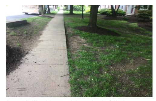
Figure 7-20 Backfill needed to prevent tripping hazard on edge of sidewalk.
