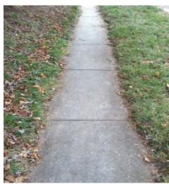
Figure 2-4 Example of a non-compliant sidewalk (less than 4ft width).
