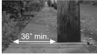
Figure 2-6 A minimum of 36" clear width is required at pinch points.
