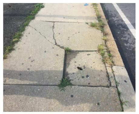
Photo 12-11 Sidewalk with multiple trip hazards.
