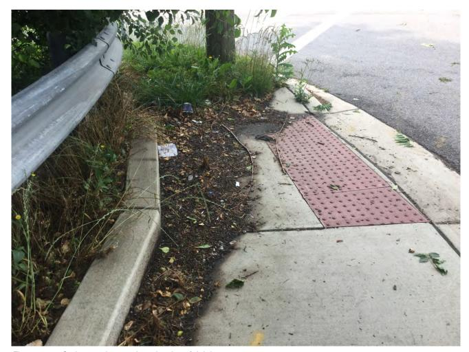
Figure 12-16 Curb ramp that requires cleaning of debris.
