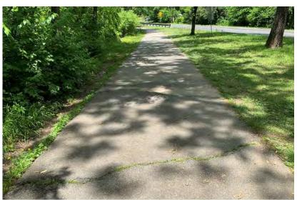
Figure 10-6 The shared-use path along Sligo Creek Parkway has some cracked or broken sections.
