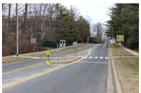
Figure 2-12 Examples of median refuges at Lockwood Drive (left) and Edison Lane (right). Install with signage to promote driver awareness (R1-16a or R1-6).
