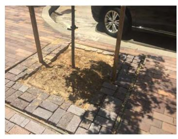
Figure 3-19 Tree pits without tree grates create tripping hazards.
