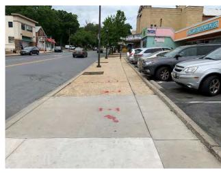
Figure 11-4 Sidewalk with non-compliant cross slope.
