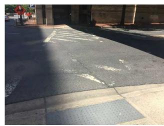
Figure 3-1 Faded crosswalk striping at Bethesda Metro Center.
