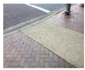
Figure 8-10 A curb ramp missing a detectable warning surface on Ellsworth Drive.
