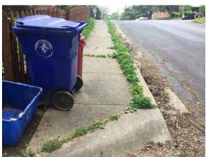
Figure 10-12 An existing sidewalk along Hartwell Road has multiple trip hazards and noncompliant slopes.
