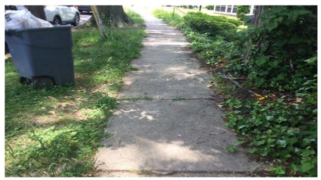
Figure 12-4 Vertical Tripping Hazard
