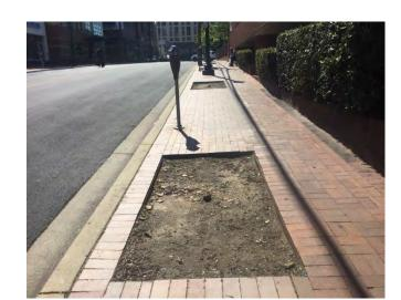
Figure 8-12 Sidewalk with multiple trip hazards
