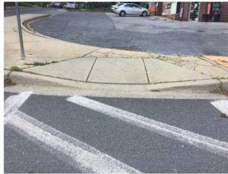
Figure 9-5 Typical non-compliant curb ramp.
