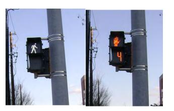
Figure 2-10 APS (left) and CPS (right) examples in Montgomery County.
