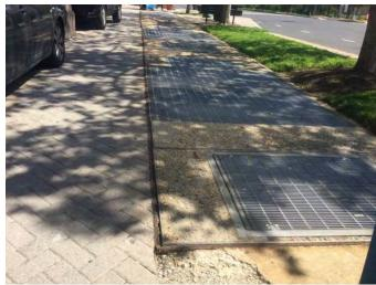
Figure 7-12 A sidewalk containing multiple tripping hazards on Wayne Avenue.
