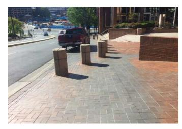
Figure 7-15 Sidewalk along Second Avenue with non-compliant slope.
