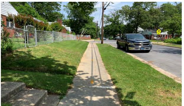
Figure 12-5 Sidewalk with non-compliant cross slope.
