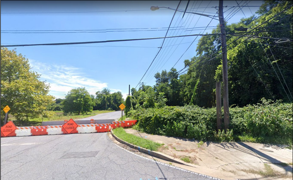
Figure 3: Closed off Area of Proposed Abandonment and Pepco Transmission Lines
