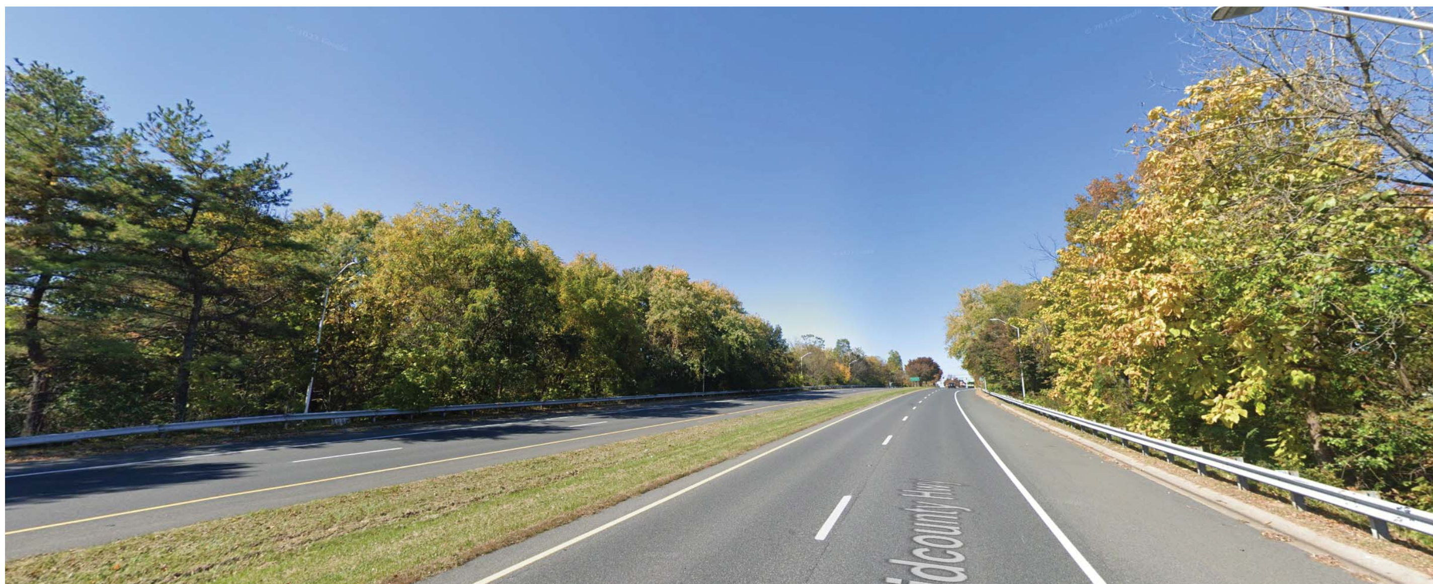
Existing Mid-County Highway (M-83) Looking North-West
