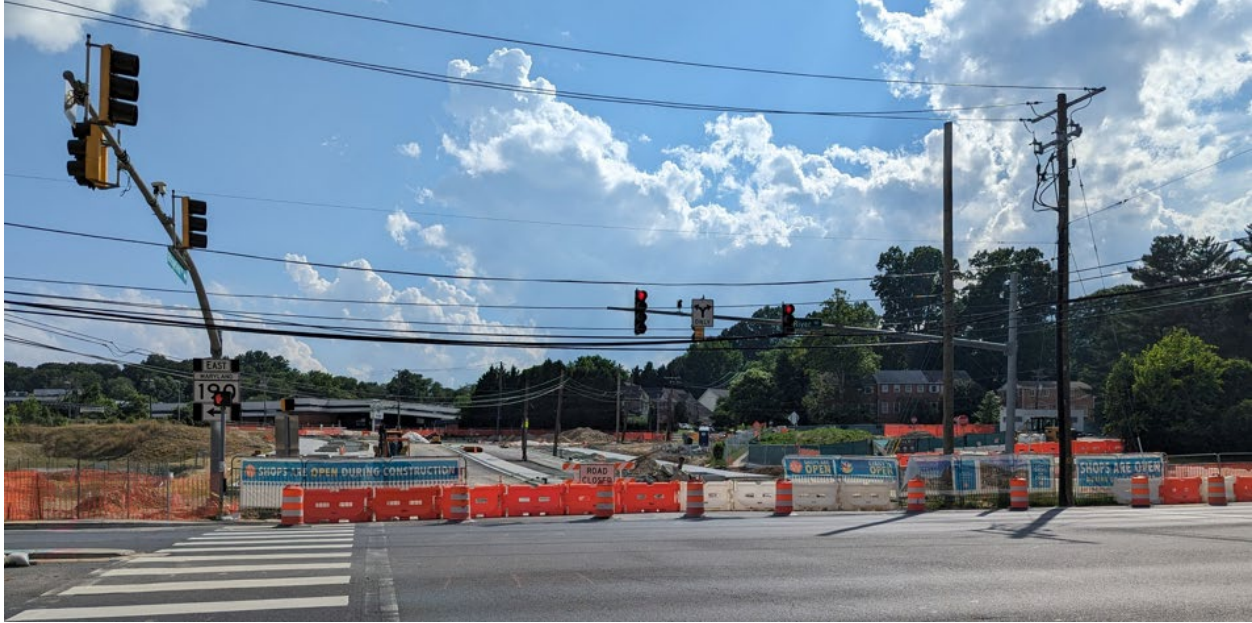
Figure 4 –Realignment Construction of Ridgefield Road Underway taken June 2023
