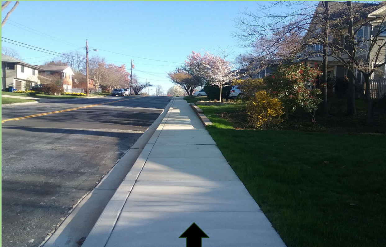
5-foot-wide concrete sidewalk at the back of curb
