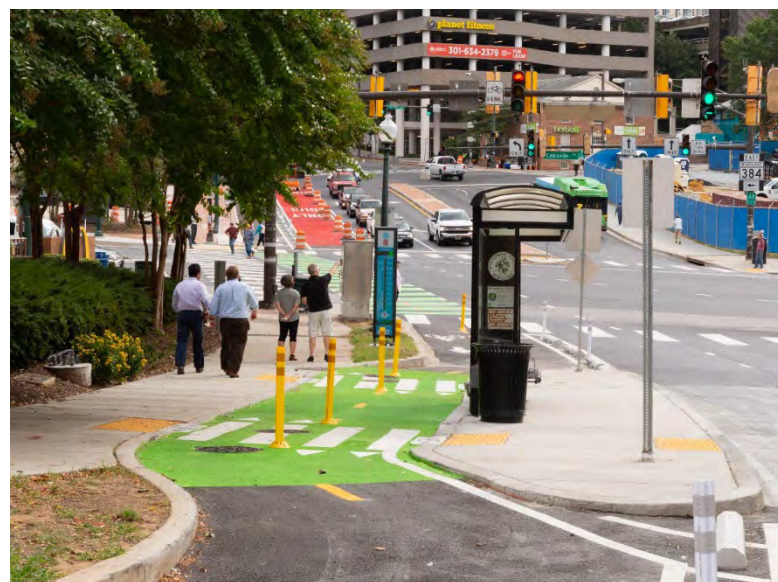
Figure 31 - Floating bus stop located at Second Avenue, north of Colesville Road, Silver Spring, MD.
