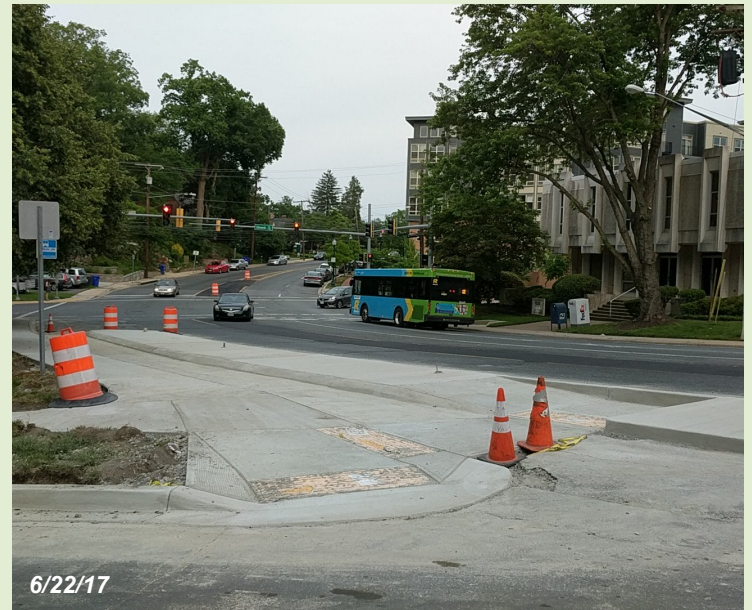
Completed floating bus stop platform along Spring Street at Ellsworth Drive. Here, the bikeway will go between the bus platform and the sidewalk, meaning the bus won't need to block the bike lane while at the stop.
