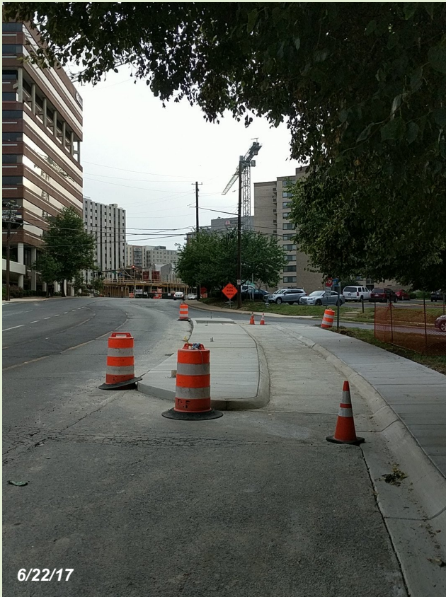
Completed floating bus stop platform along Spring Street at Ellsworth Drive. Here, the bikeway will go between the bus platform and the sidewalk, meaning the bus won't need to block the bike lane while at the stop.
