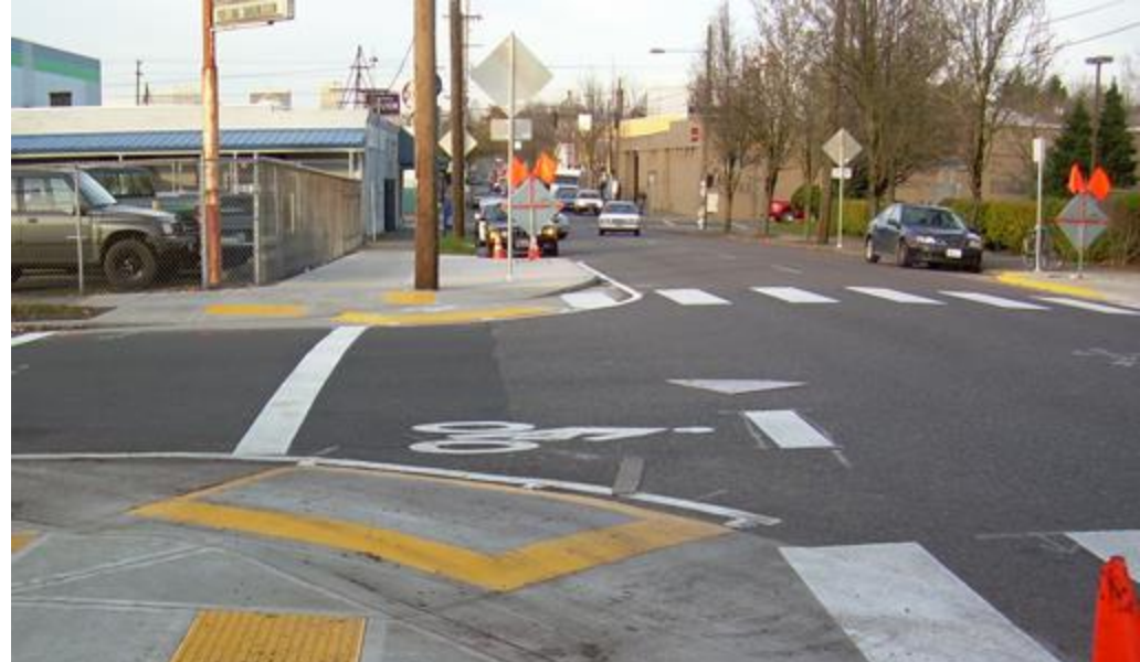
Intersection Improvements – Bicycle Forward Stop Bars Image Source: NACTO
