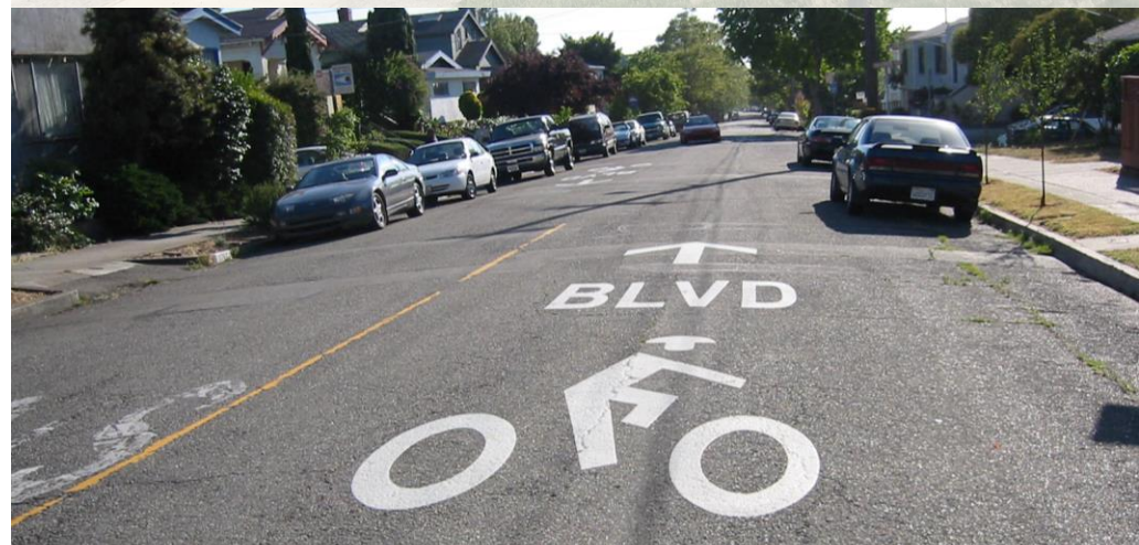
Bicycle Boulevard Pavement Marking Image Source: NACTO
