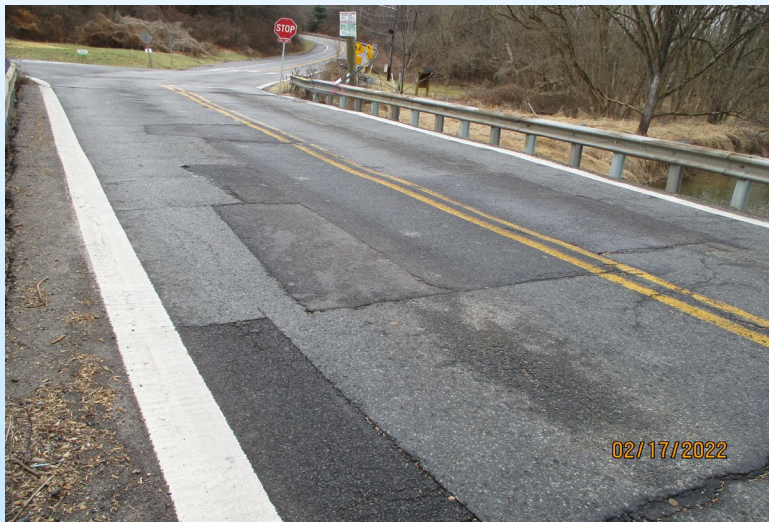
Asphalt Patches
