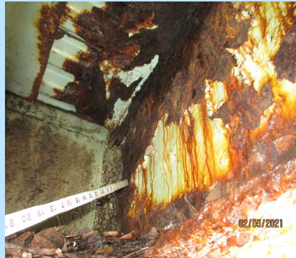
Peeling Paint, Rust Staining and Heavy Corrosion at Beams
