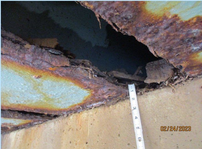
Peeling Paint, Rust Staining and Heavy Corrosion at Beams
