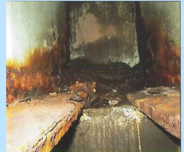
Heavy Corrosion and Section Losses
