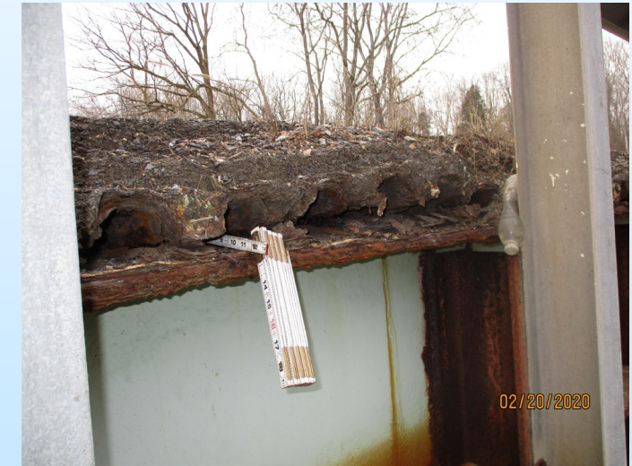
Severe Corrosion to SIP Form
