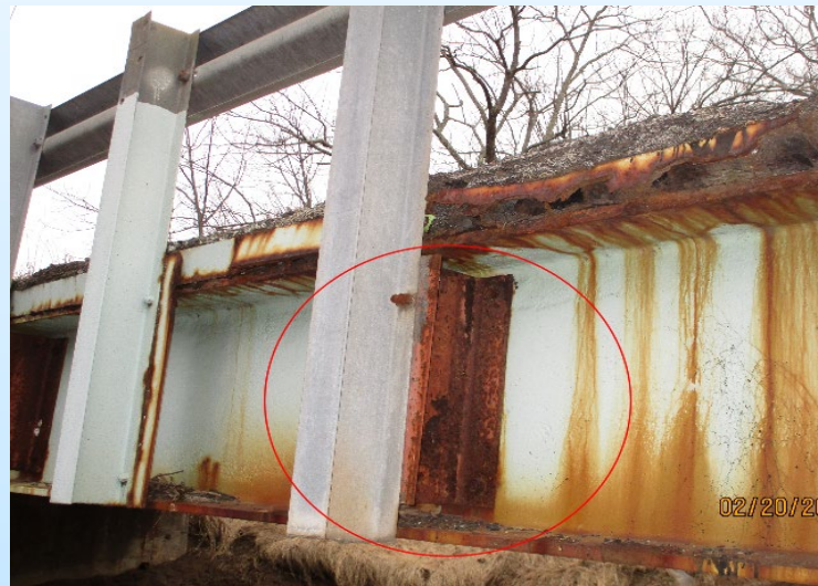
Railing Post Connection Corrosion
