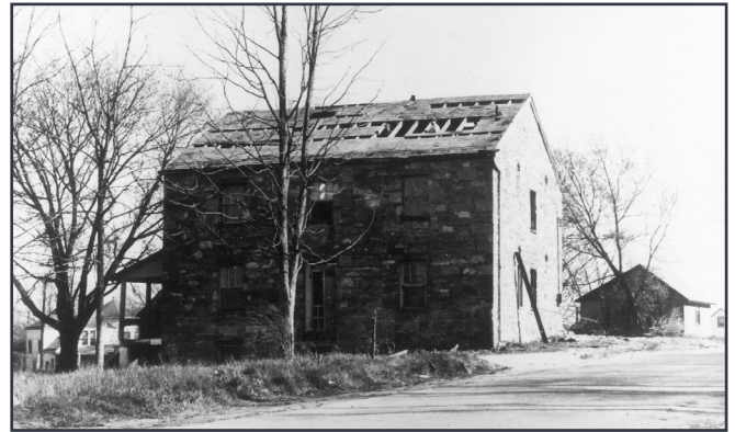
The Rockville jail building, located on the property where the County Council Office Building stands today. Taken c. 1932 just before its demolition. ( Montgomery History )
