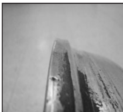
Photo 9. Sharp edge removed.
