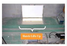
Have the rescuer exit the working and then close the doors using the wheel on the door operator. Close the hoistway doors and while standing in the middle of the car top, push the direction button to move the elevator into position next to the stalled car. Open the emergency hatch of the stalled car, and, using a folding ladder, rescue any trapped individuals.
