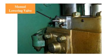
First, using lock-out/tag-out, ensure that the power has been shut off and place a firefighter at the lower hoistway opening with the doors open. Open the valve at the top of the car until the elevator moves. When the car reaches the same level as that of the firefighter at the lower hoistway, close the valve. This will stop the elevator and allow access for the rescue.
