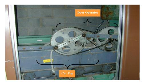
Hoistway doors provide protection for the hoistway opening. They may be single speed or two speed horizontal, bi-parting vertical, or swinging. Swinging doors are normally found on residential elevators. The doors operator will open the car doors which will then allow access to the passengers. The car doors are the only doors that are powered.
