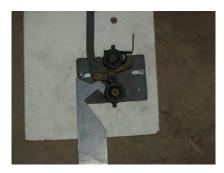
If poling the elevator is necessary, use the hook and access from the closest door using the appropriate elevator key. Using the pole, unlock the hoistway door above. Additional personnel stationed at the elevator above will open up those doors, pull up the pole and utilize that pole to open the door above.
