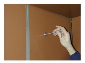
Once the key drops through the backside of the car door, turn the key until it catches on the pick-up roller arm. Continue to turn key until car door opens.
