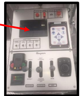
Aerial Information Center on the Pedestal Control Panel
